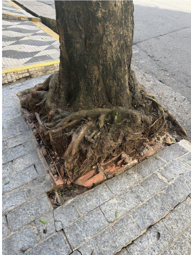
Plate 2. Exposed buttress and surface roots overflowing a sub-meter pit, with brick and mortar infill marking prior pavement repair work.
