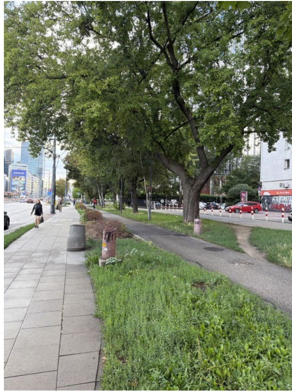
Plate W-3. Continuous unpaved vegetated verge — no cut pit. Effectively unrestricted lateral soil volume and a permeable surface. Note the flexible asphalt path threading past the trees.
