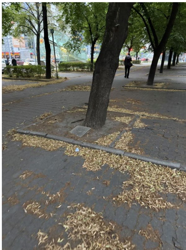
Plate W-1. Mature linden in an undersized pit cut into monolithic paving. Note the perforated aeration/irrigation plate set into the pit surface — evidence of designed accommodation — and the constrained, near-flush root flare.
